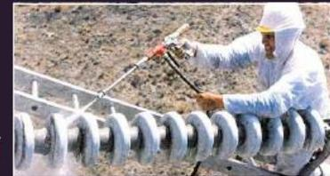
Ash is cleaned from a 220 kV strain insulator string using pressurized water following the 1995 Ruapehu eruption, New Zealand (Transpower New Zealand)
