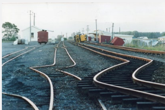
Substation and railway damage from the Edgcumbe earthquake. Source: Archives New Zealand
