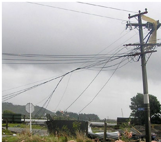
Damaged powerlines. Source: National Emergency Management Agency
