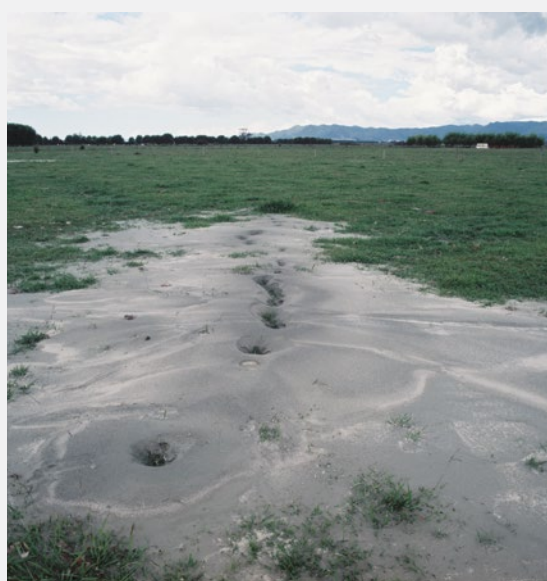
Sand boils and liquefaction after 1987 Edgecumbe Earthquake. Source: GNS Science Photographer: Lloyd Homer
