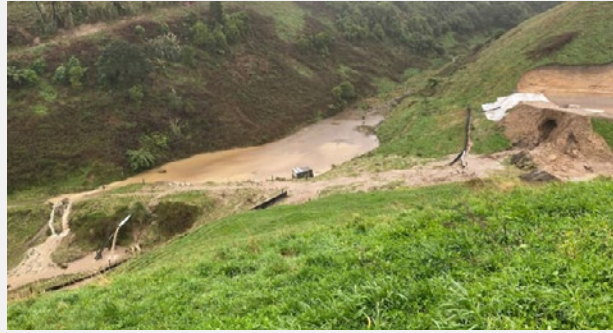
Sediment-laden water discharging from a hole in a sediment retention pond and flowing over land at a kiwifruit development property in 2022. Source: Newstalk ZB
