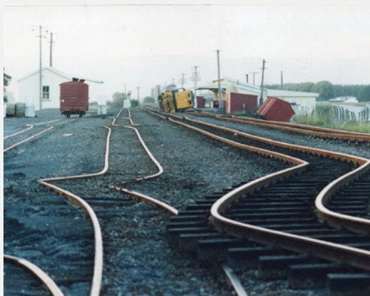
Damage to Railway lines, Edgecumbe. Source: Archives New Zealand, CC BY-SA 2.0
