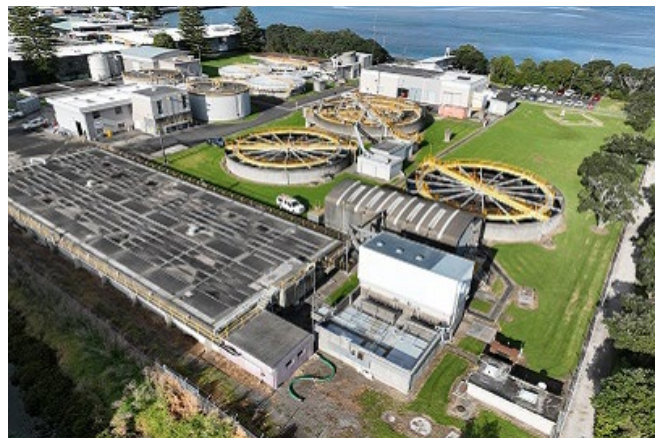
Chapel Street treatment plant. Source: Tauranga City Council
