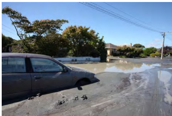
Extensive and severe liquefaction, Christchurch.
