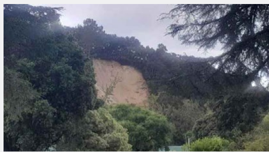
Slip | Council land behind Tamarangi Drive, Kawerau. Source: Rotorua Daily Post
