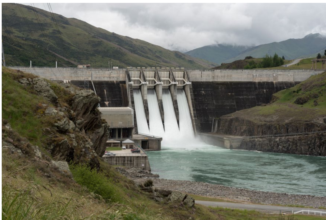
The Clyde hydroelectric power dam spilling large amounts of excess water – Clyde, Otago. Source: Adobe Stock
