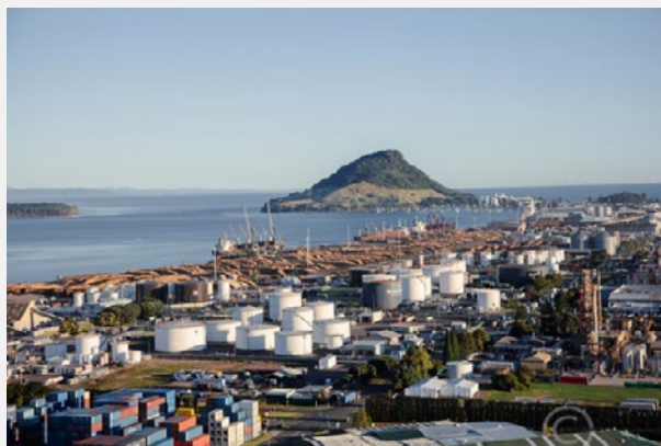
Mount Maunganui Industrial Zone. Source: Bay of Plenty Regional Council
