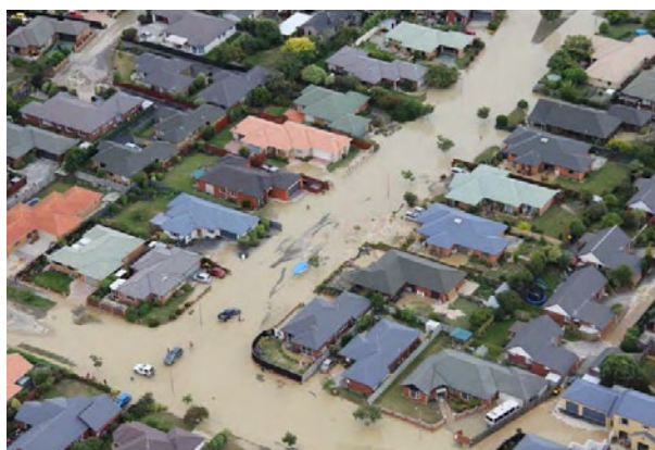
Extensive and severe liquefaction, Christchurch.
