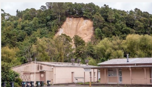
Slip | Council land behind Tamarangi Drive, Kawerau. Source: Sunlive
