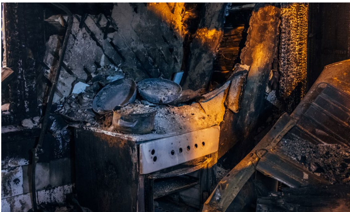
Burnt house interior. Source: Adobe Stock
